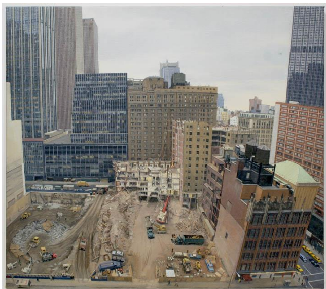
Demolition and Excavation on the Site of the Equitable Life Assurance Society's New Tower at 7th Avenue and 52nd Street, 1983. Oil on Canvas, 32 x 36 in.
